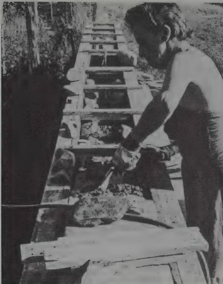
Helen building the stone wall around the garden in Maine, late 1960s.
